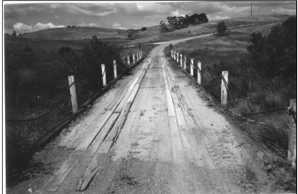
Typical Timber Bridge
